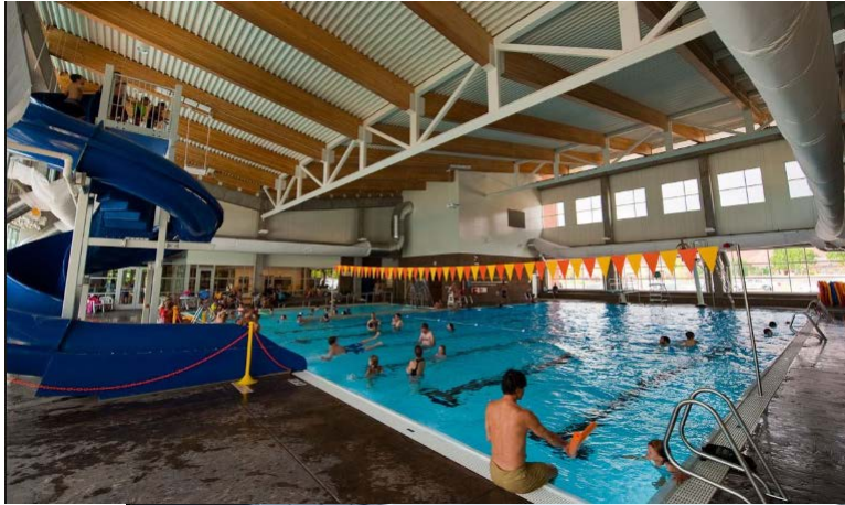
Moab, UT (50,000 SF + outdoor leisure pool)
