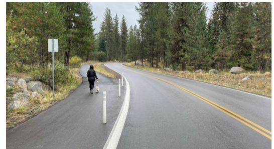
Pathways alongside roads with no curbing require some type of detectable edge between the pathway and the street.
